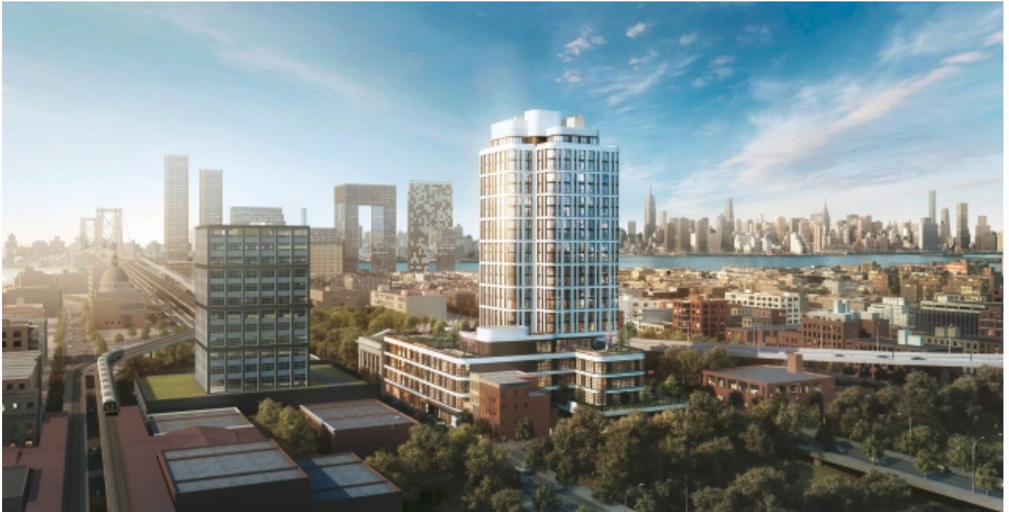
A VIEW OF THE DIME FACING MIDTOWN AND THE UNDER-CONSTRUCTION DOMINO SUGAR FACTORY DEVELOPMENT. RENDERING: FOGARTY FINGER ARCHITECTURE
